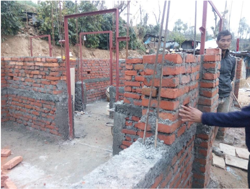
Brick masonry in cement mortar with concrete band
