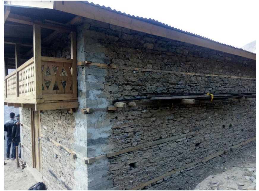
Stone masonry in mud mortar with wooden band
