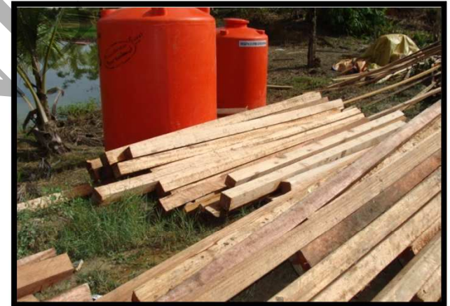
3. Stock Material Shelter
