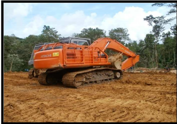
1. Land clearing shelter area
