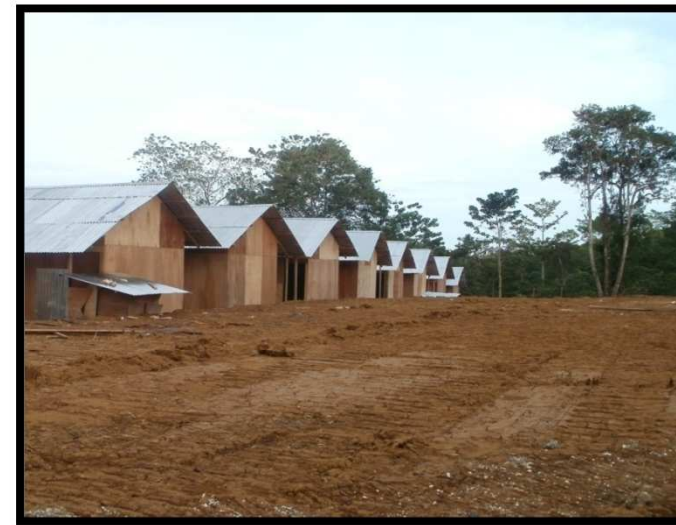
Shelter KM 10 North Pagai
