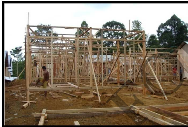
4. Erection Frame shelter
