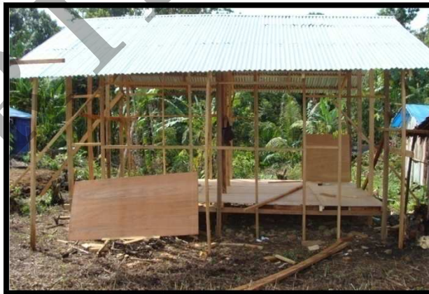
5. assembly roof and wall
