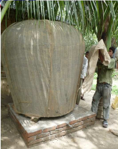
Initial stage of construction of RWH unit
