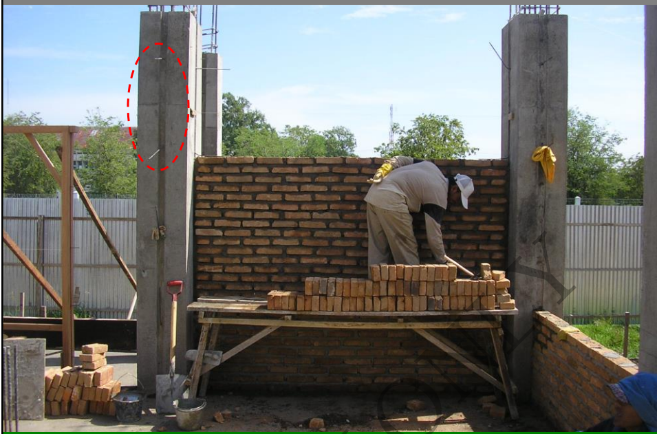
NURSING COLLEGE, UNSYIAH, ACEH WALL TIES BETWEEN COLUMNS AND WALL
