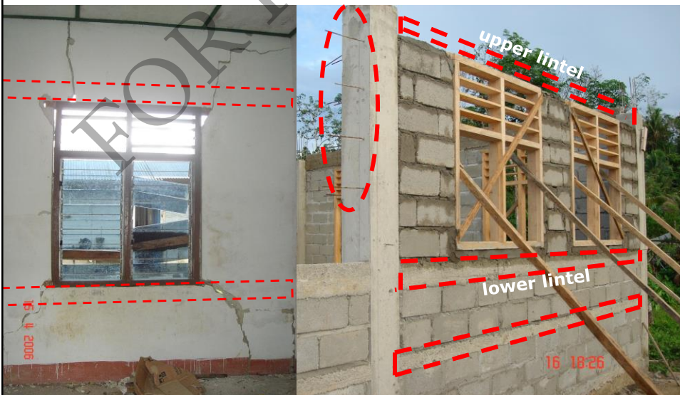
PUSKESMAS PLUS AWAAI POTENTIAL CRACKING AREA ON WALL &amp; OPENING – DOUBLE LINTEL
