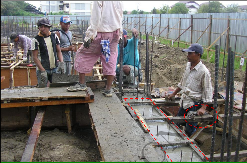
NURSING COLLEGE, UNSYIAH, ACEH EXTRA ANCHORAGE SYSTEM FOR GROUND BEAMS
