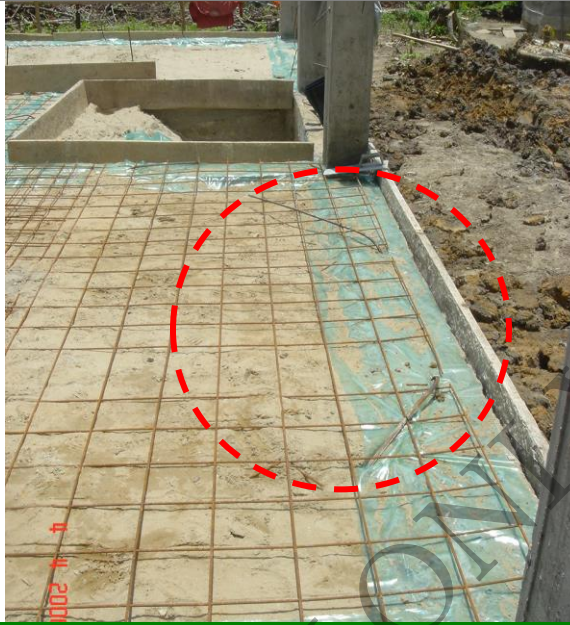
PUSKESMAS PLUS AWAAI STEEL LAPPING BETWEEN BRC AND GROUND BEAM
