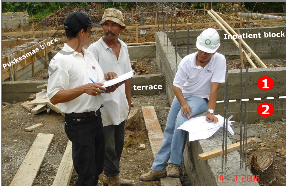
PUSKESMAS PLUS AWAAI DOUBLE BEAM - SEGREGATION OF BLOCK
