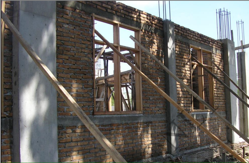
NURSING COLLEGE, UNSYIAH, ACEH DOUBLE LINTELS AT OPENING
