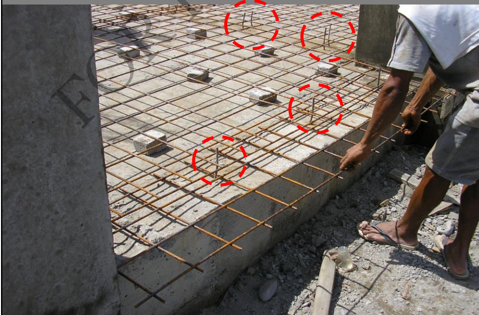
NURSING COLLEGE, UNSYIAH, ACEH FLOOR SLAB REINFORCEMENT BAR AND ANCHORAGE
