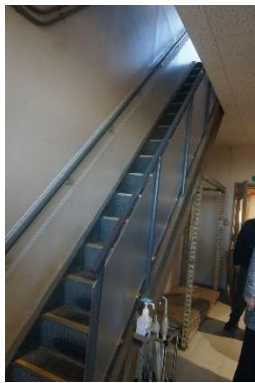
(e)全校師生用此樓梯爬至三樓避難
