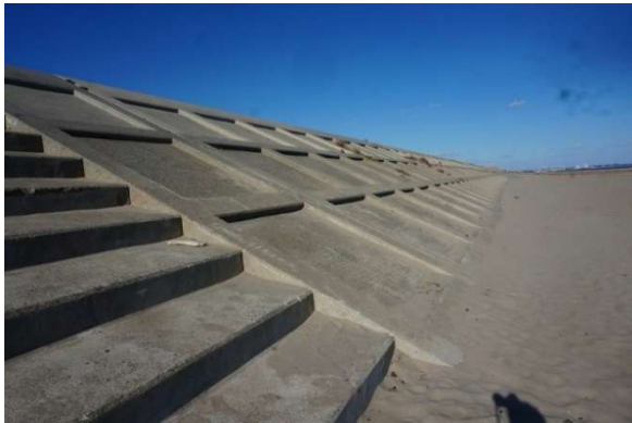
(c)海岸堤防(靠海側)及階梯
